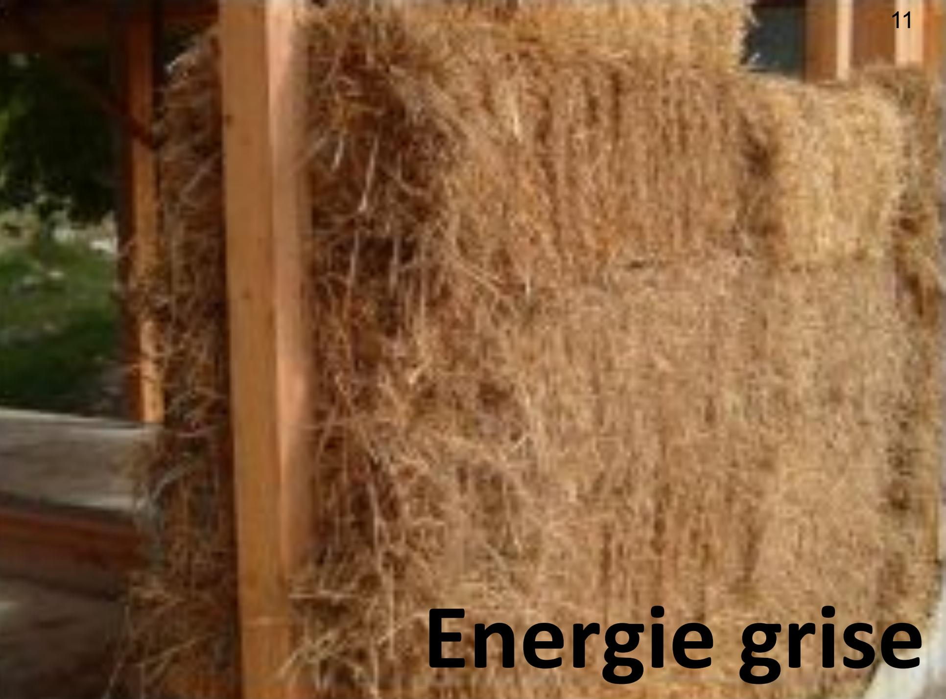
A close-up photograph showing a wooden frame structure filled with straw insulation. The straw is light brown and fibrous, packed between vertical wooden studs. The background shows a blurred outdoor scene with green foliage.
